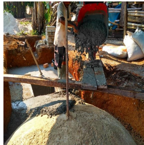
Gambar 6. Proses Pengecoran Digester
