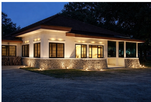
Figure 1. Doterswoning House View
