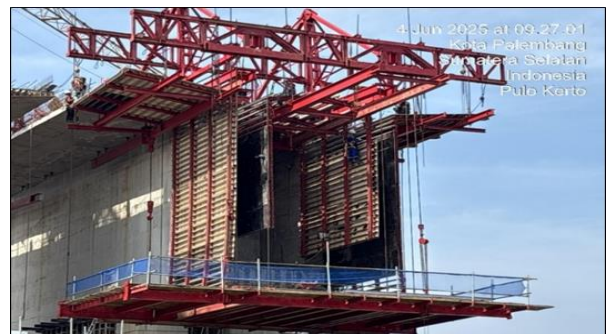
Gambar 4. Proses Instalasi Segmental Box Girder Proyek Musi V
