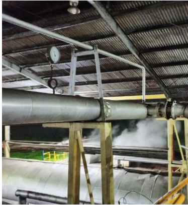
Gambar 3. Pipa Line Steam Back Pressure Vessel ke Sterilizer
